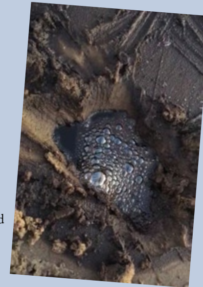
Becker Well in Leaking Form (Photo by Nora McNeely Hurley)
