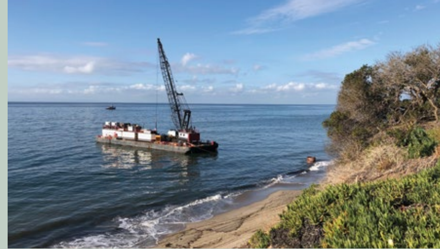
The giant barge from Curtin Maritime, Long Beach, is towed into Summerland Beach in front of Becker Well, and drops a giant pipe onto the beach. This "cofferdam" is hammered into the sand around the well and pumped clear of sand and water to create a work space. The work platform is lowered on top of the cofferdam so that workers can descend to the top of the well and do their magic.
