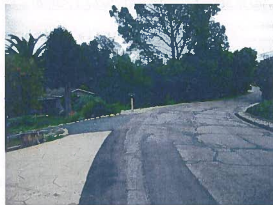
FIGURE 4. LA ENTRADA, LOOKING EAST
