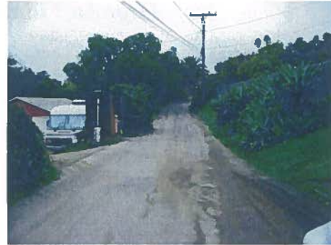
FIGURE 2. VISTA VALLEJO, LOOKING NORTH
